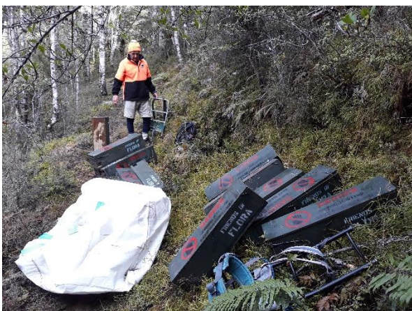
Mike at work on TK line
